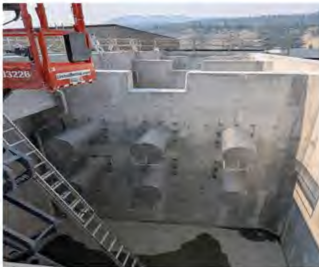
Photo 4: MBBR Sieves Install
