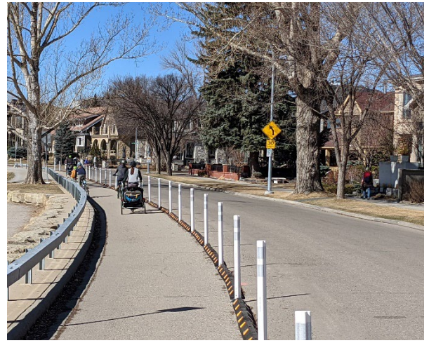
Example of a quick-build MUP in Calgary, AB using rubber barrier curb and plastic delineators
