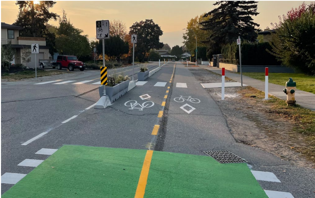
An additional quick-build example WATT Consulting designed in Kelowna, BC.
