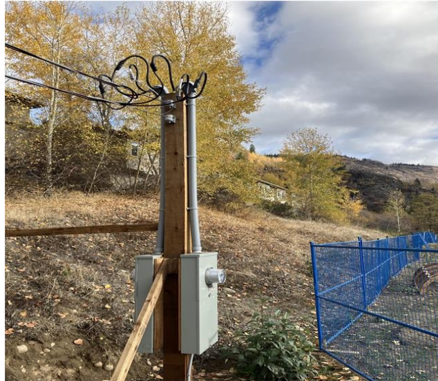
Photo 2: Fortis Temp power install North Yard
