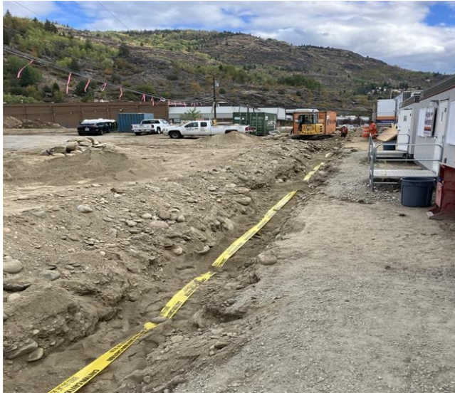
Photo 1: Install NG Line
