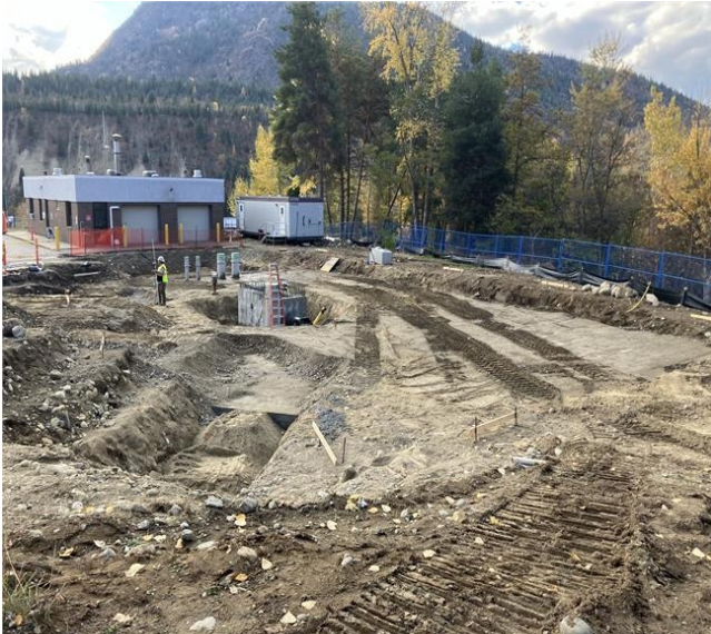
Photo 7: Backfill and Prep HW Subgrade
