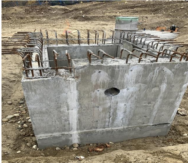
Photo 6: Headworks Sump Stripped and Prepped for Leak Test
