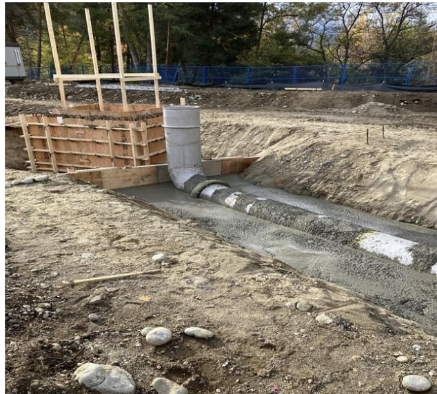
Photo 4: 600mm SRS Pipe Encasement
