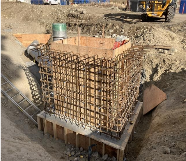
Photo 5: Form and Reinforce Headworks Sump
