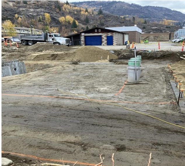
Photo 8: Headworks Footing Prep
