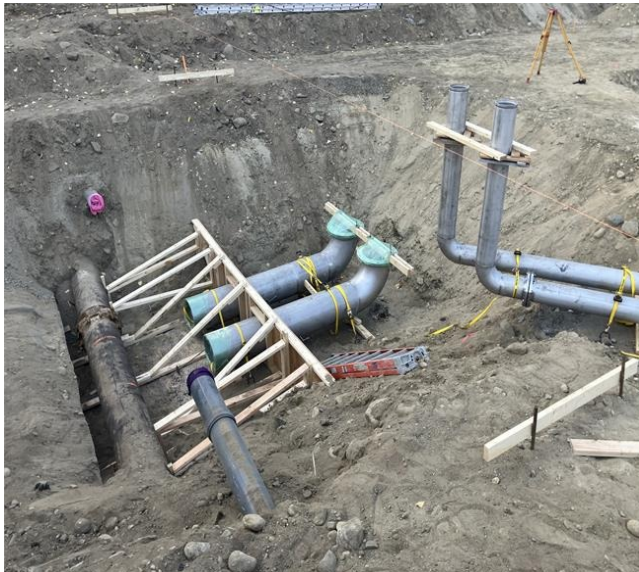
Photo 3: Install and Test HW Under Slab Process Piping
