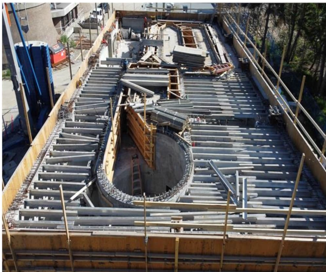
Photo 1: Headworks El. 433.00 Slab Shoring
