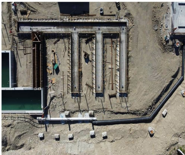
Photo 4: Buried 600mm ML HDPE & SS Install
