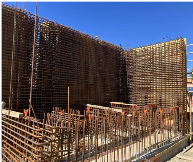
Photo 2: MBBR Splitter Box Walls Rebar
