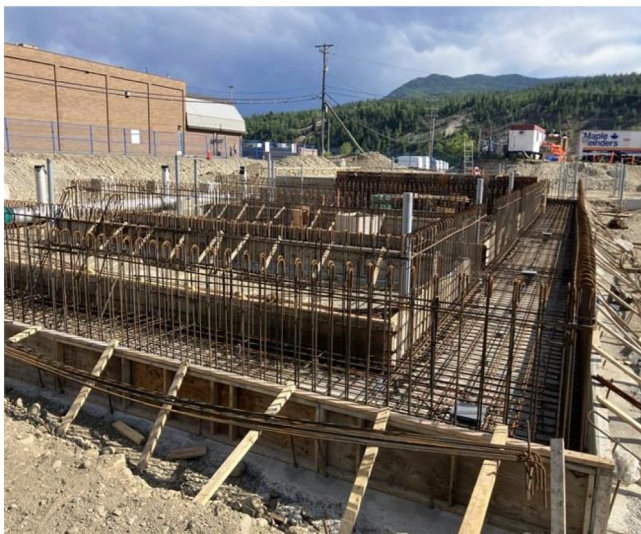
Photo 3: DAF Pipe Channel Slab and Walls Underway
