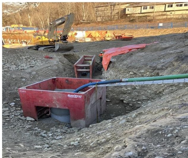
Photo 4: SMH 5C installation and By-pass
