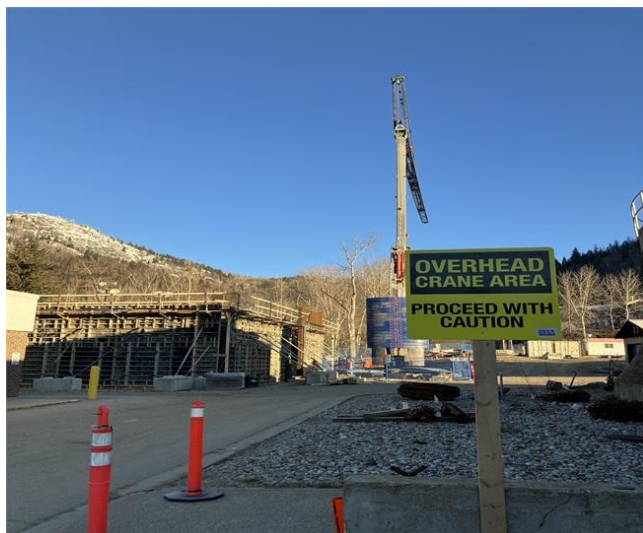
Photo 3: Headworks Building with Self-Erect Crane
