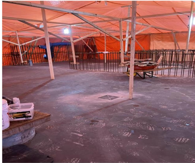
Photo 2: Headworks Base Slab
