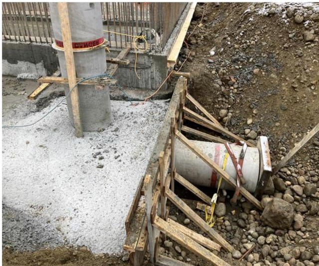
Photo 3: 600mm ML Pipe Install
