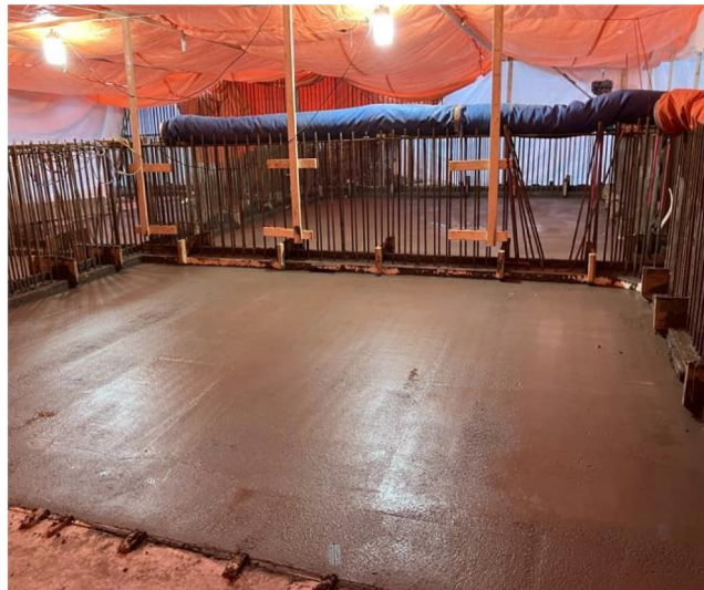
Photo 4: MBBR Base Slab Pours 3 and 4
