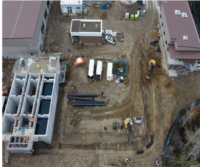
Photo 2: Install of SRS line and leaktesting of MBBR
