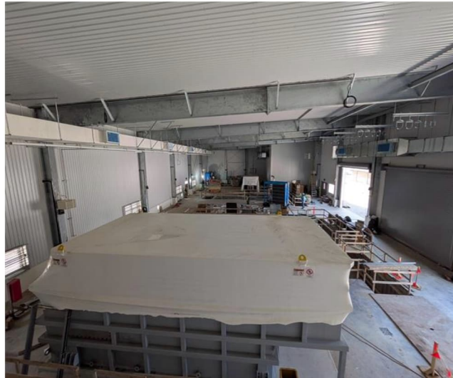
Photo 4: DAF building from mezzanine. HEX install underway.
