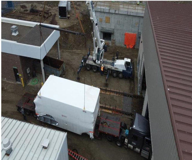
Photo 3: DAF Clarifier #1 lifted and skated into the building
