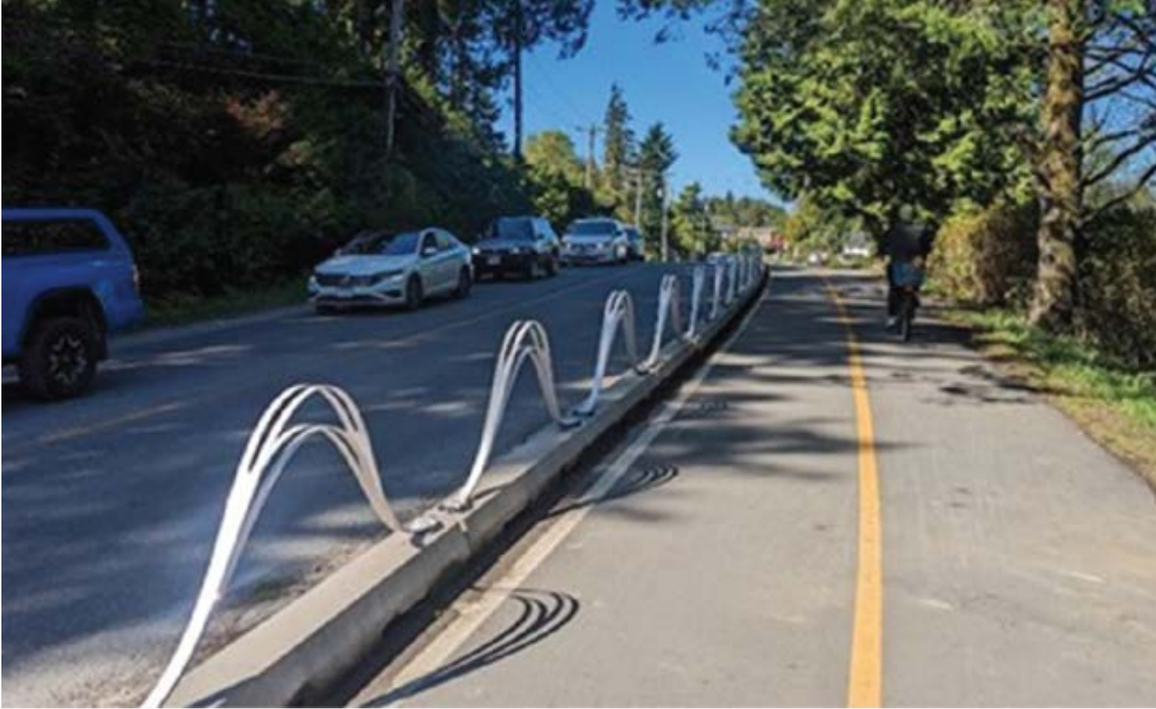
Separated Multi-Use Pathway with Barrier
