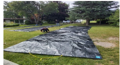
Figure 15: Floating Benthic Mats Laid Out
