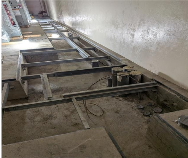
Photo 2: DAF Electrical MCC Supports Installed
