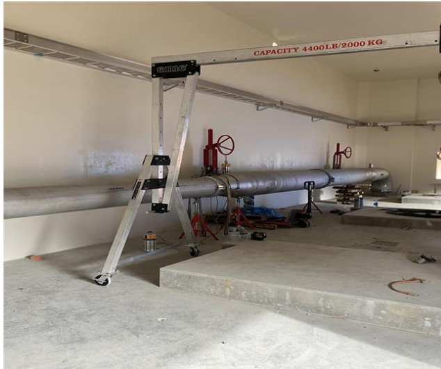
Photo 4: ML Pipe Installed
