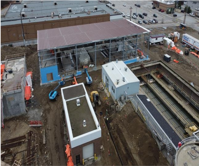
Photo 1: DAF Pre-Eng Underway
