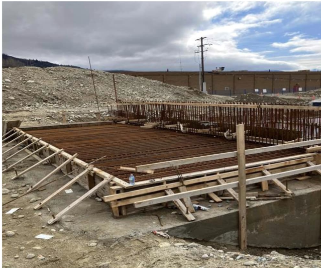
Photo 3: MBBR Splitter Box Base Slab
