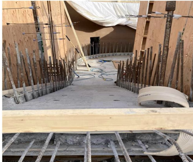
Photo 4: Headworks Grit Vortex
