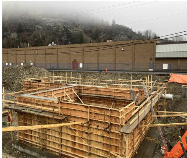
Photo 2: DAF Final Effluent Wet Well and Reclaimed Water Clear Well Walls
