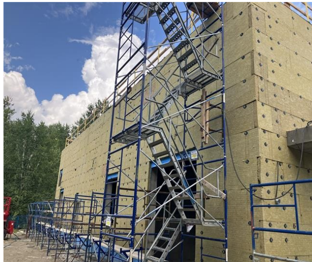
Photo 4: Headworks exterior insulation
