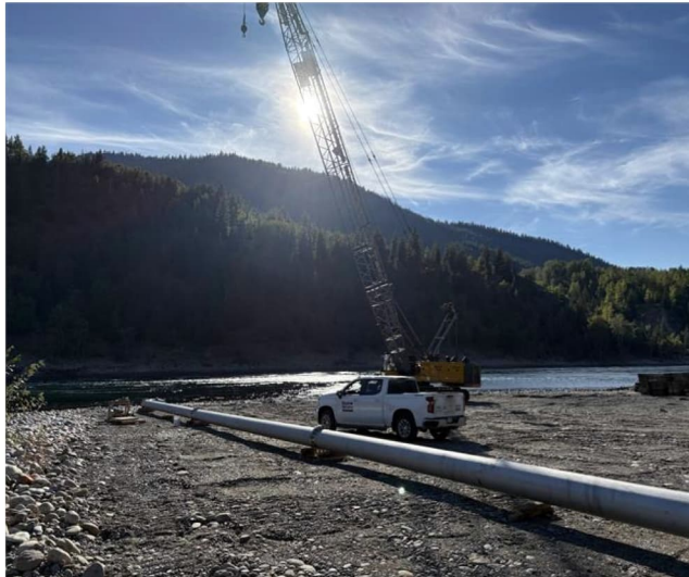
Photo 4: Outfall Pipe Bolted Up
