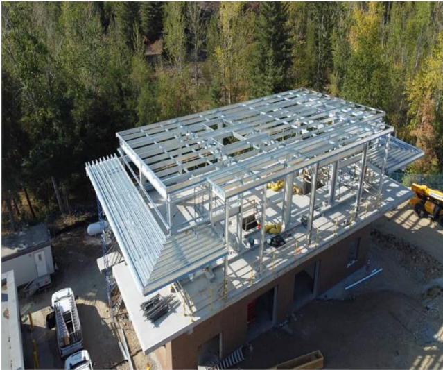
Photo 1: Headworks Pre-eng building
