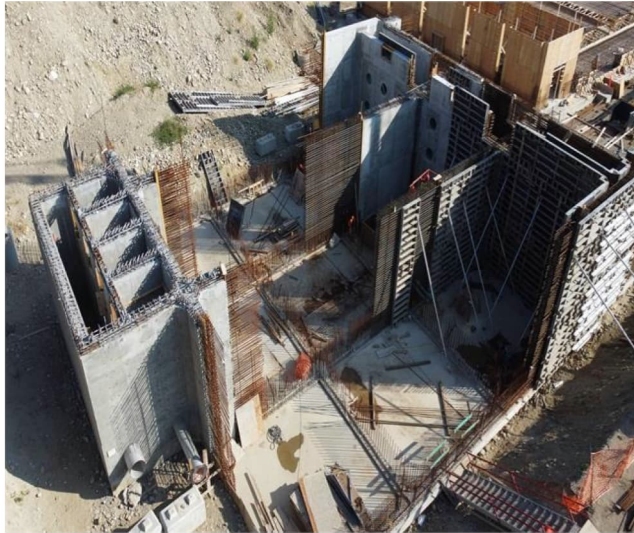
Photo 2: MBBR Southern Walls Poured
