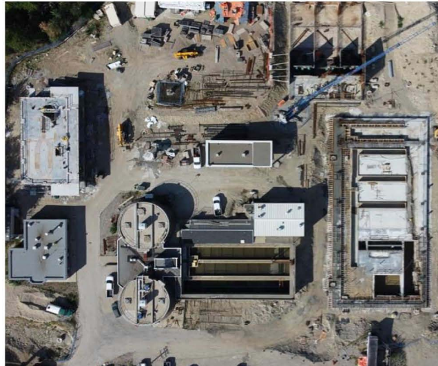
Photo 4: Overall photo of site
