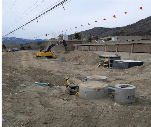
Photo 2: DAF Pump Station Backfilling and Manholes
