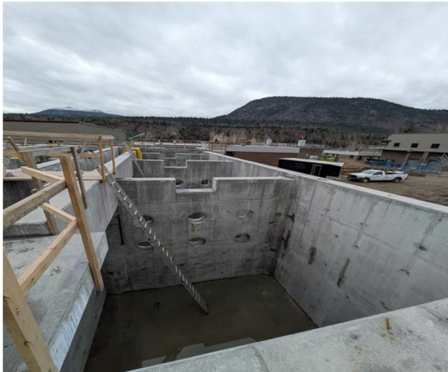
Photo 3: MBBR Train 1 Ground and Patched
