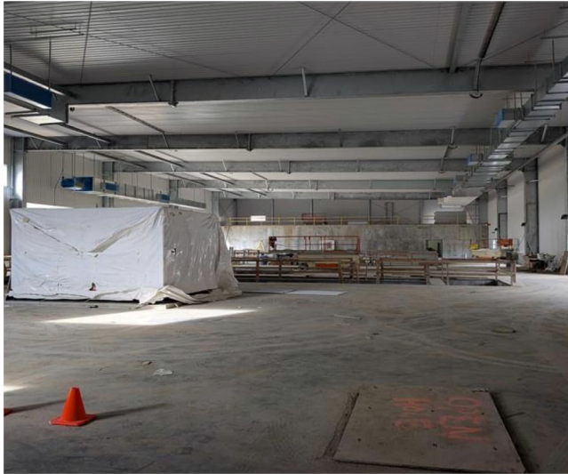
Photo 1: DAF Pre-eng Complete and Ducting Underway
